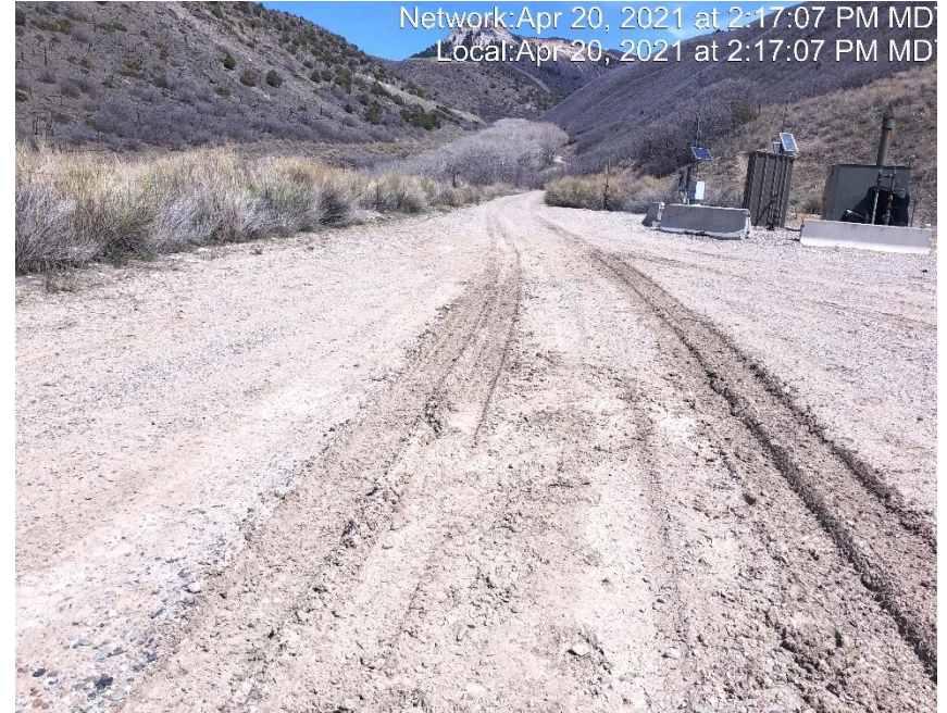
Photo #3563 No form of tracking BMP at entrance to location.
