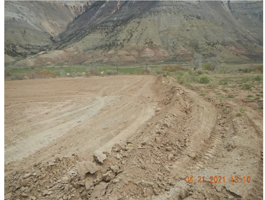
Uncompacted berm
