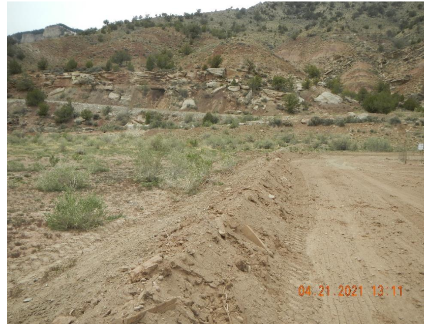
Trash and debris bladed into uncompacted berm.
