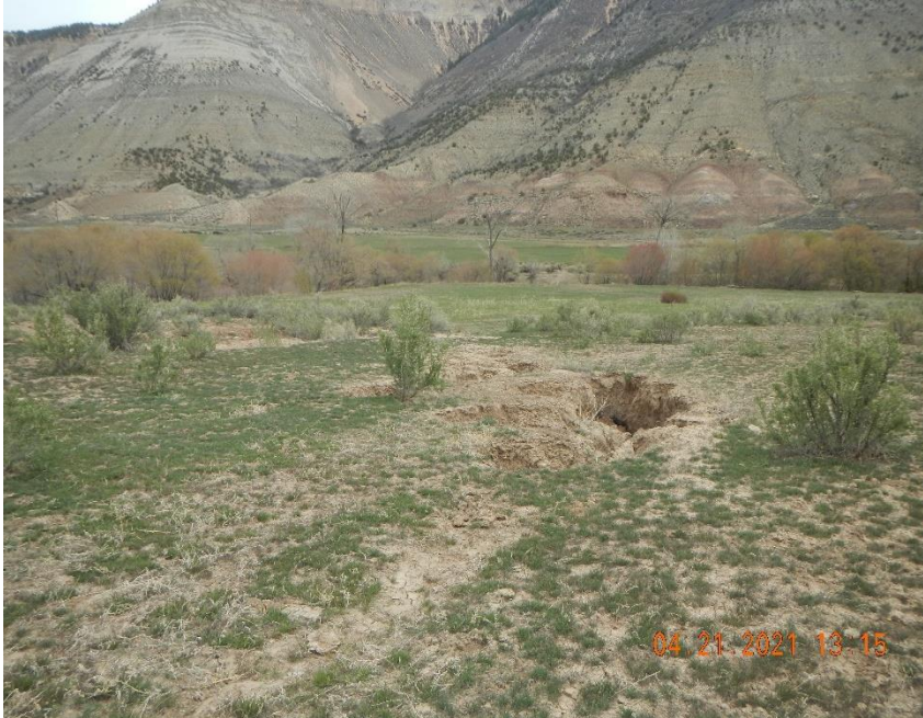
Erosion channeling down path of location drainage.
