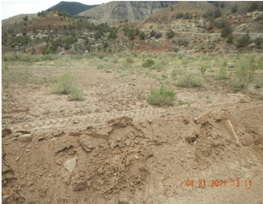
Trash and debris bladed into uncompacted berm.
