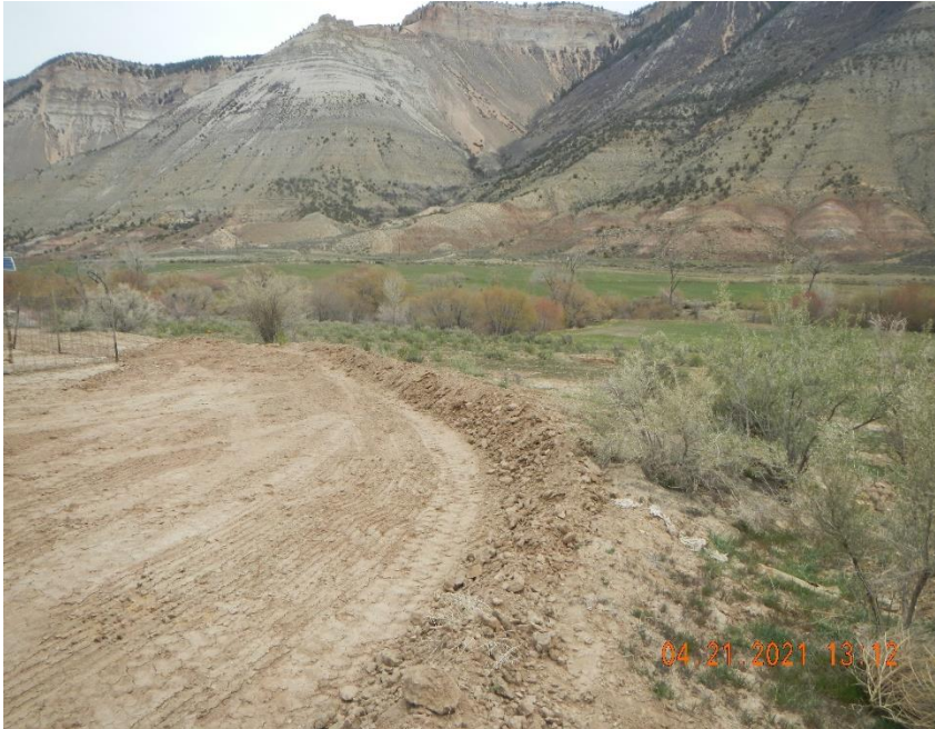
Uncompacted berm.
