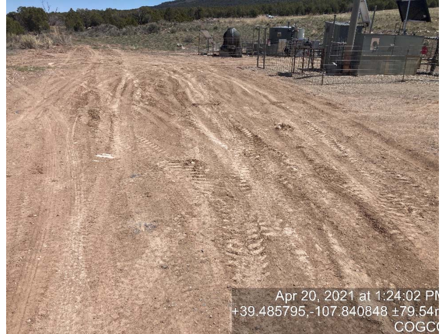
lack of stabilization/compaction
