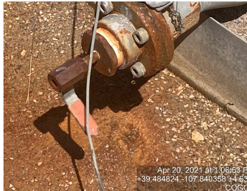
Tank valve leaking
