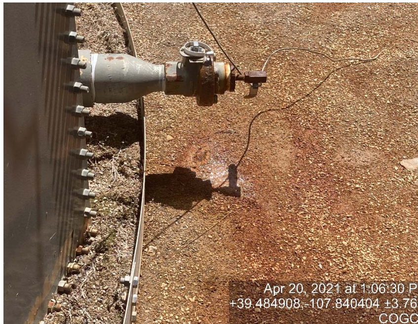
Tank valve leaking
