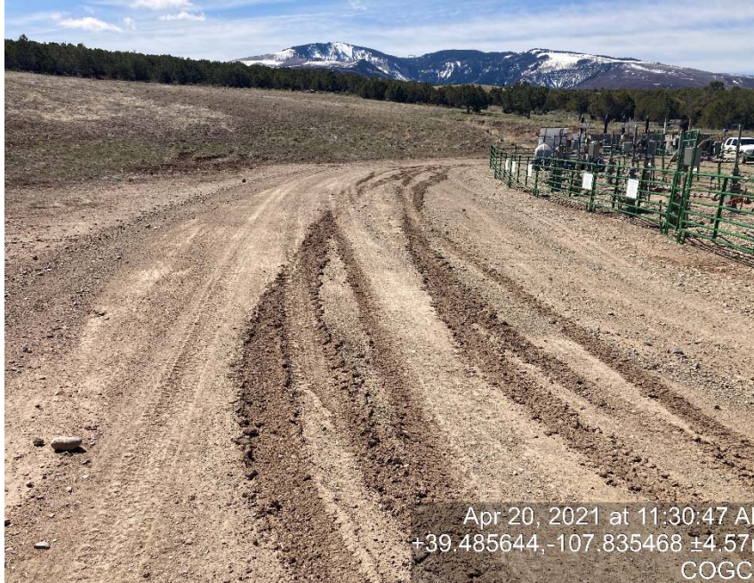
Lack of stabilization/compaction
