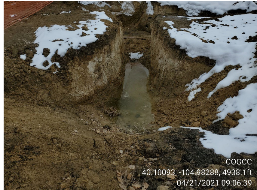
Photo 5: Excavation at flowline release. Water is presumed to be stormwater.
