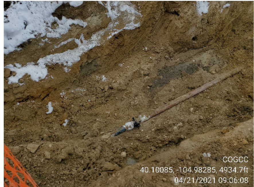
Photo 3: Excavation of release and flowline repair.
