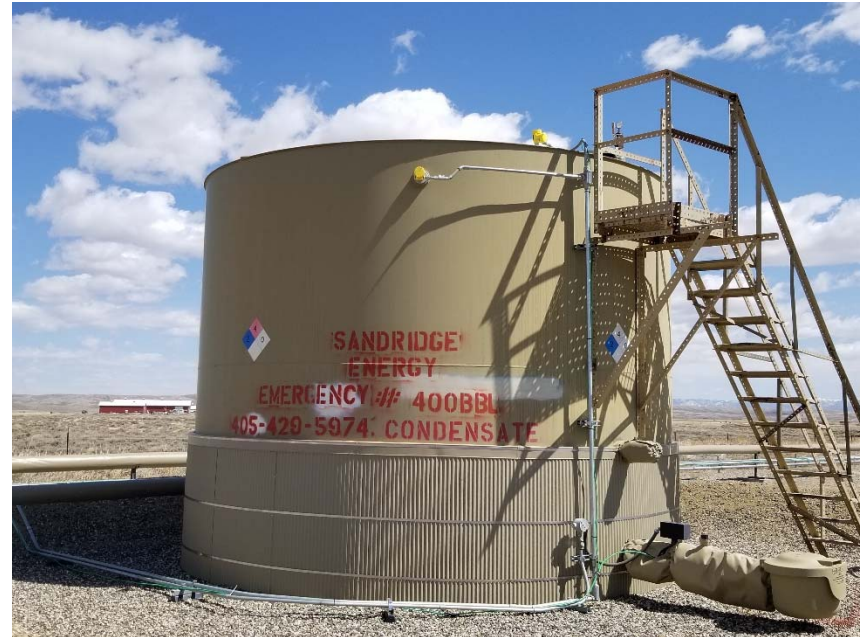
Photo 7. Incomplete/inaccurate tank label.
