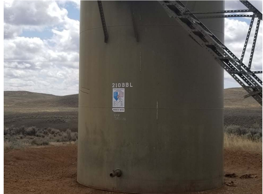
Photo 2. Incomplete/inaccurate tank label.
