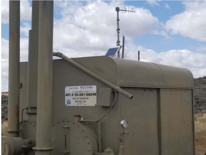
Photo 1. Battery sign at separator not battery. Sign is incomplete/inaccurate.
