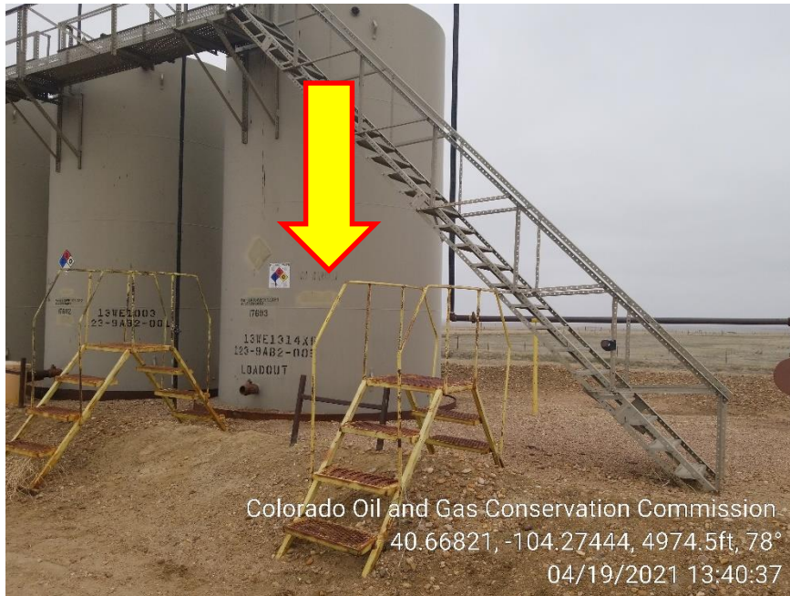
Photo 3 – H2O Tank – Capacity Label fading
