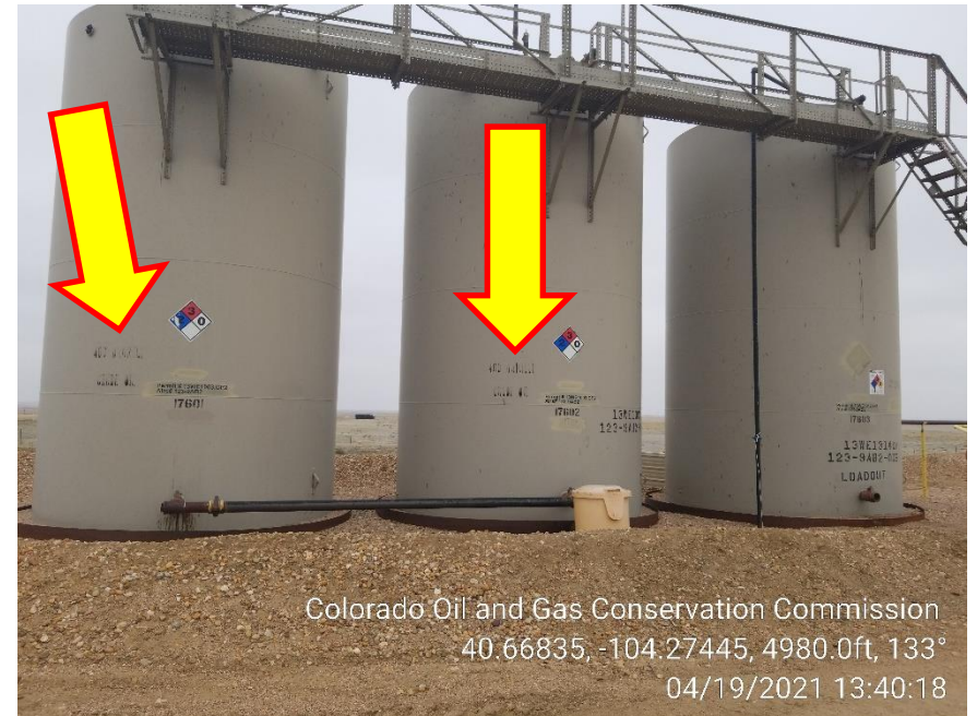
Photo 2 – Crude Oil Tanks – Capacity and Content Labels are fading
