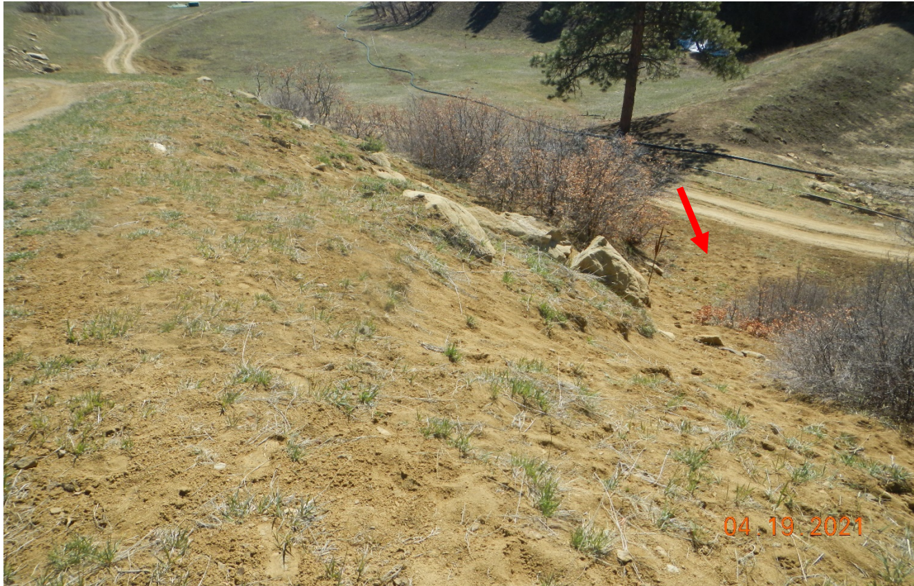
Photo 3. Facing toward the fill slope of the road. There is sediment deposition in area shown at red arrow from erosion of the fill slope.
