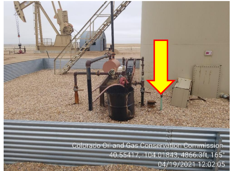
Photo 4 – Unmarked Riser
