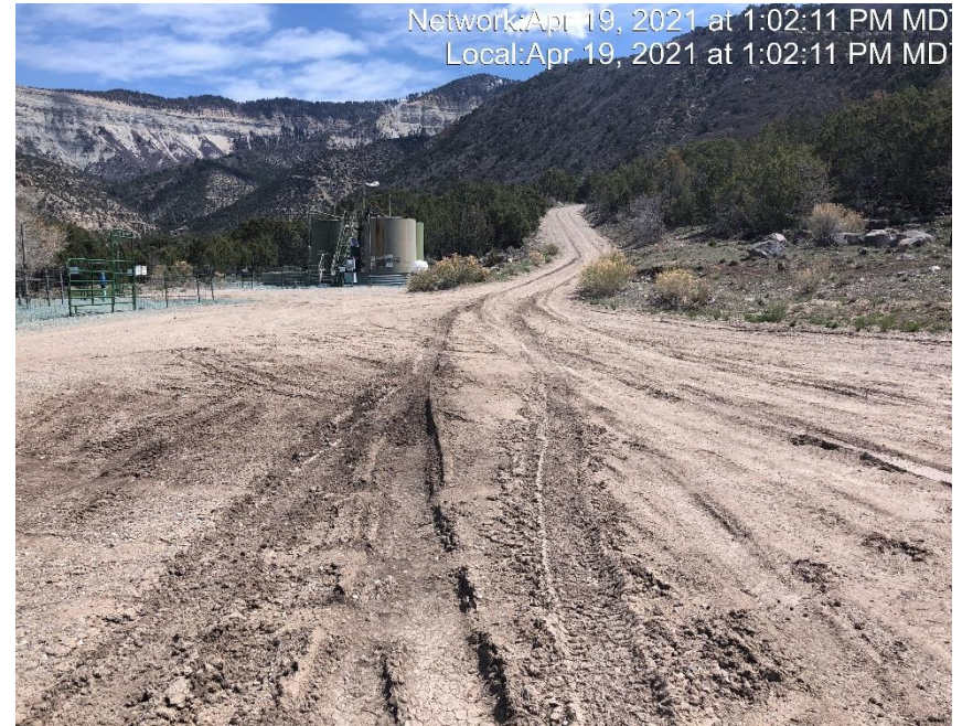
Photo #3538 No form of tracking control at entrance to location.
