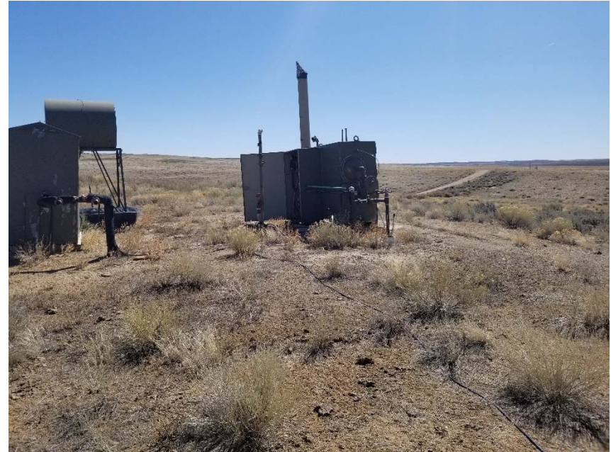
Photo 3. Unmarked risers at separator.
