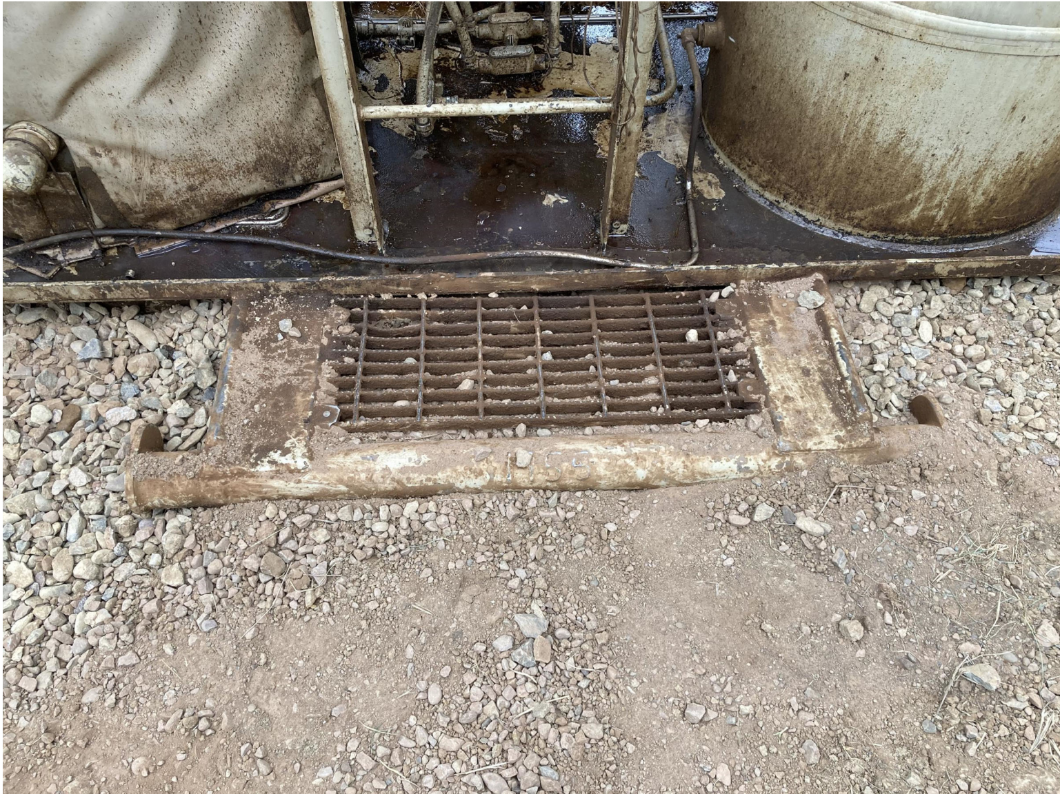
PHOTO 1: THE OIL ACCUMULATION ON THE SKID OF THE SCREW COMPRESSOR WAS REMOVED AND THE IMPACTED SOIL ON THE GROUND WAS CLEANED UP.
