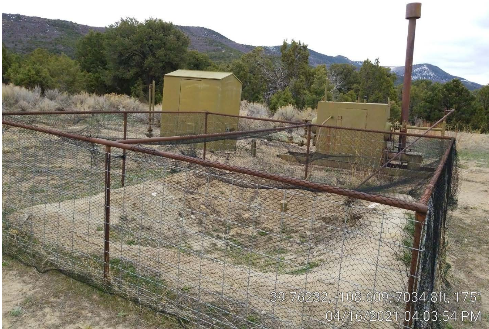
Photo 3. Pit, meter building, separator.
