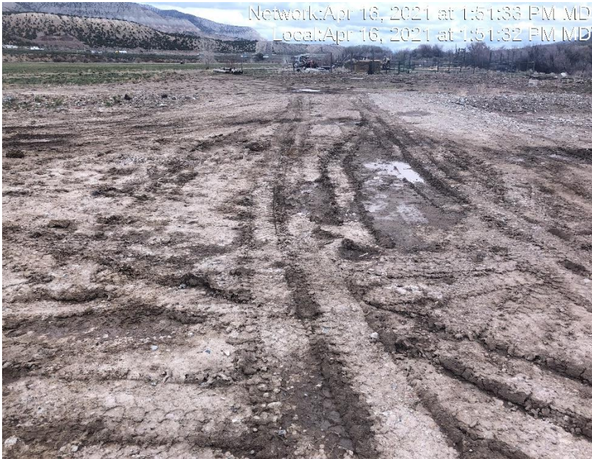
Photo #3528 No form of tracking control at entrance to location.
