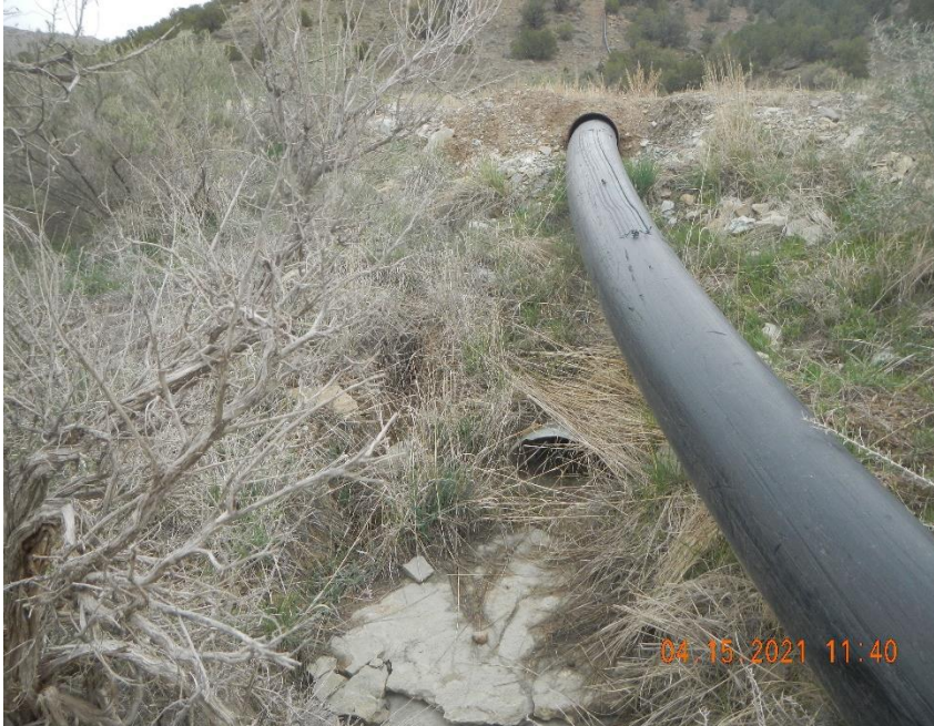
Culvert outlet needs cleaned.
