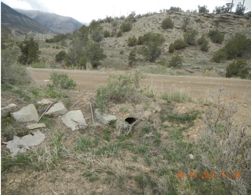
Inlet basin of culvert needs cleaned out.
