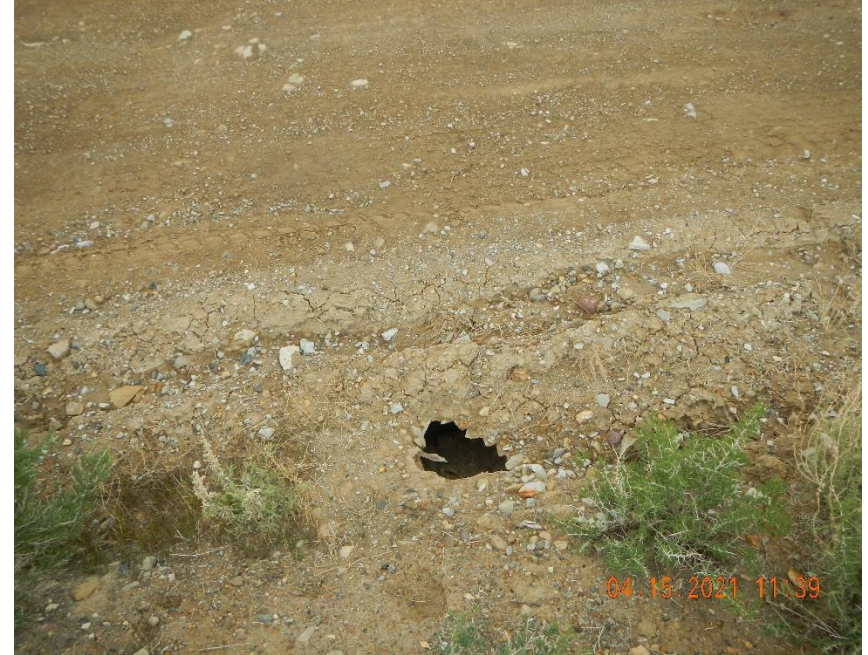
Culvert is damaged in road side ditch.
