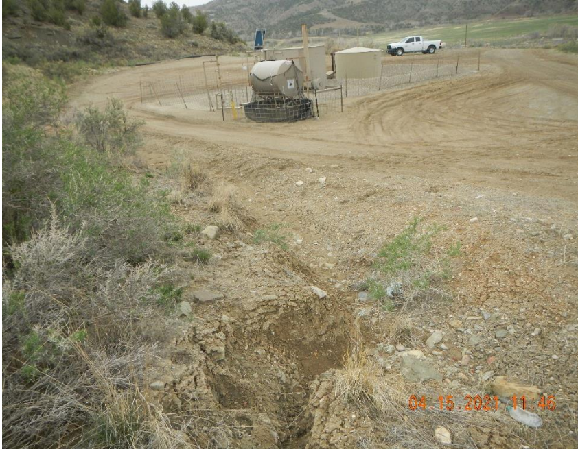
Storm water damage on perimeter ditch around location.
