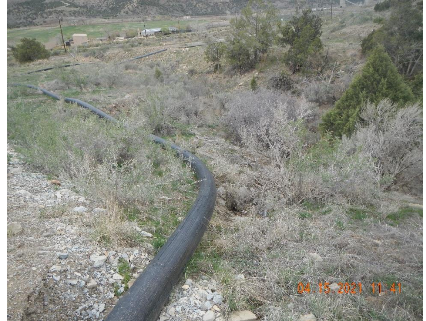
Storm water washing bank at culvert outlet.
