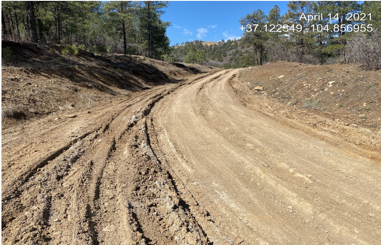
Photo 3. There is vehicle rutting along the first switch back in the road. It appears vehicles are spinning out in this area.
