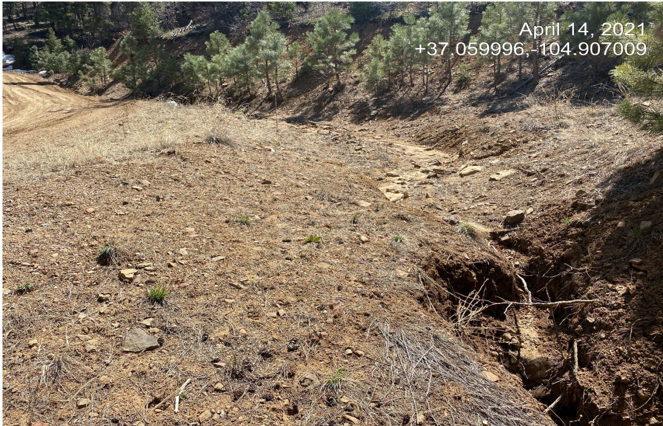
Photo 4. At the second switch back in the road, stormwater diverted off the road has caused erosion in bottom right of photo. This area needs to be stabilized with BMP's
