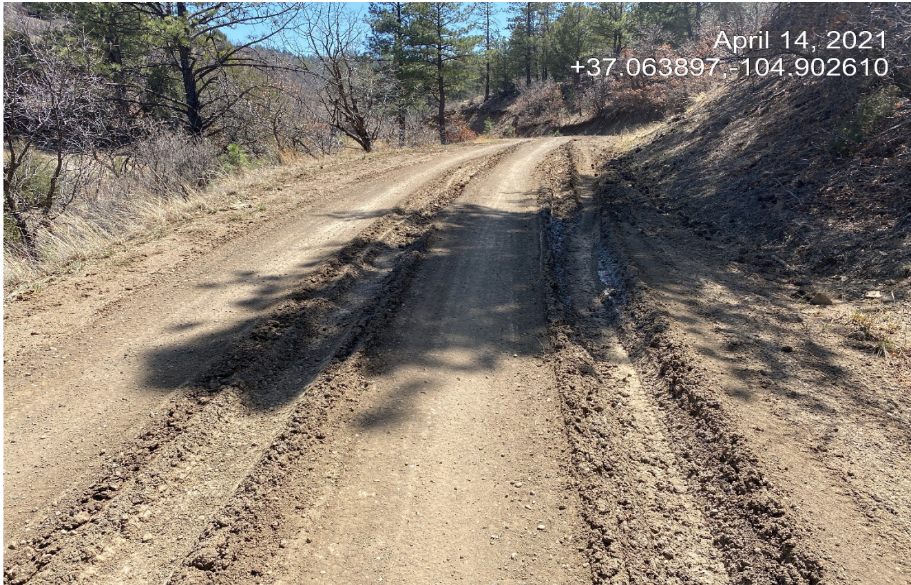
Photo 2. There are vehicle ruts along areas of the road which need to be repaired and stabilized.
