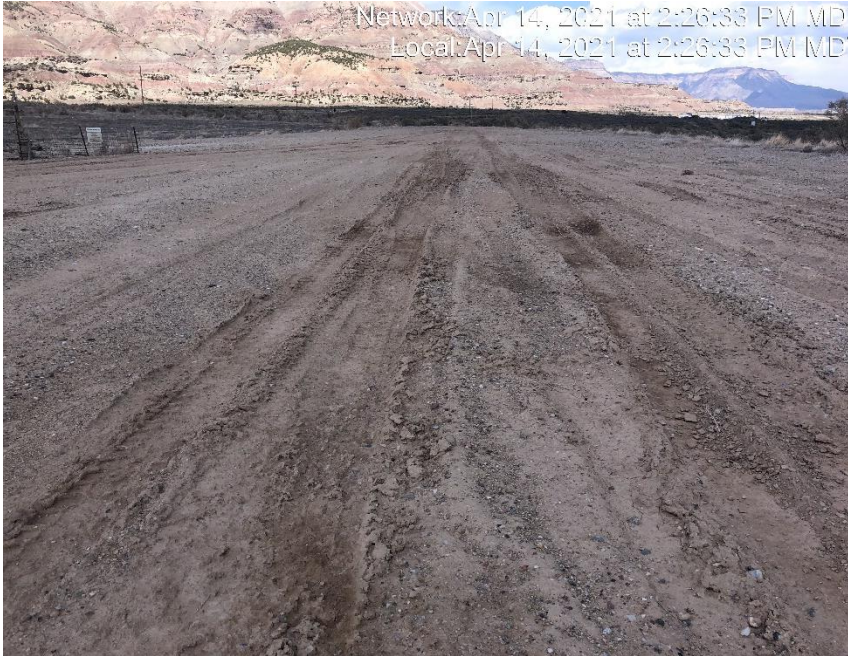
Photo #3492 Location lacks stabilization.
