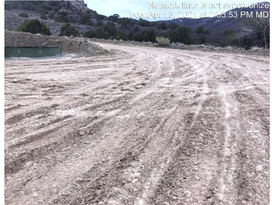
Photo #3480 No form of tracking control at entrance to location
