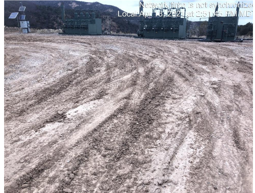
Photo #3478 Location lacks stabilization.
