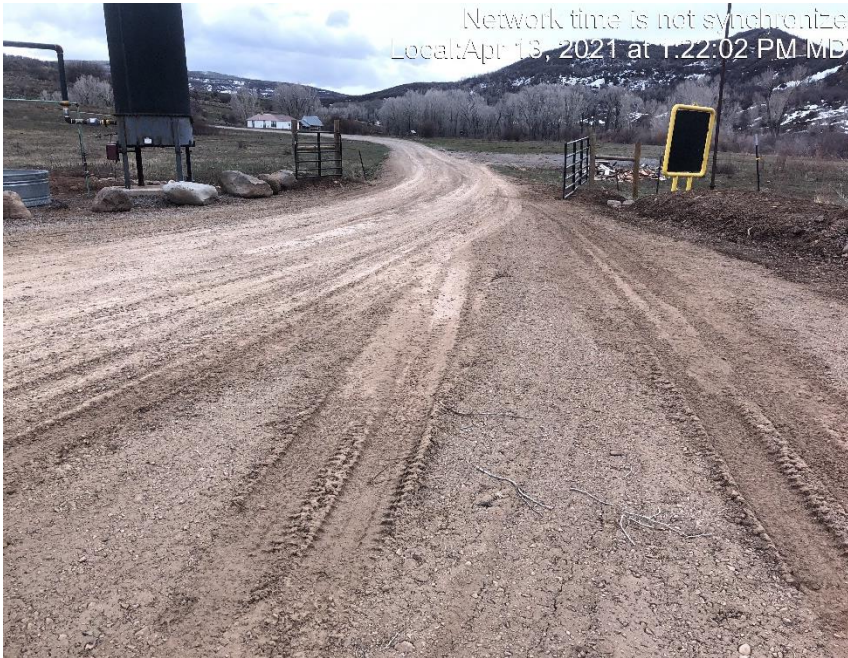
Photo #3470 No form of tracking control at entrance to location.
