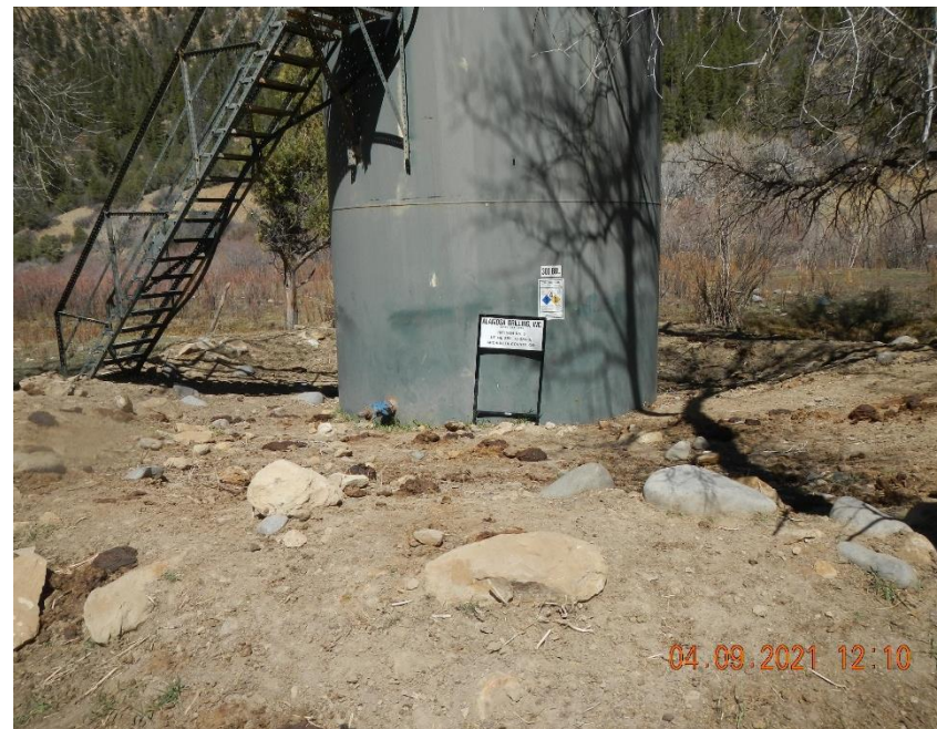
Nielson #5 crude oil AST. Tank battery sign is not compliant with Rule 605.e(2). Secondary containment does not appear to have adequate capacity.
