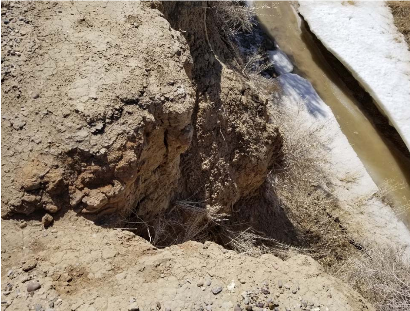
Photo 7. Erosion rills transporting sediment off location.
