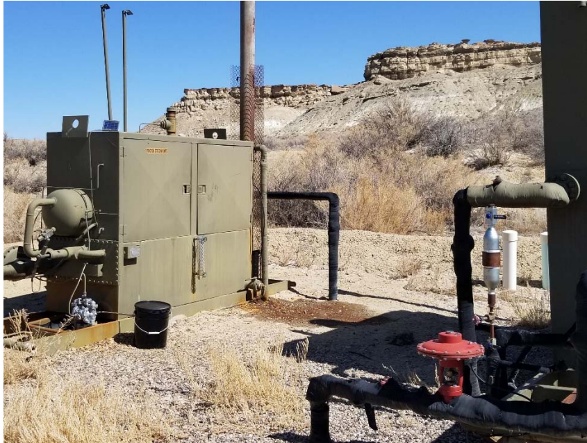
Photo 3. Stained soil at separator.
