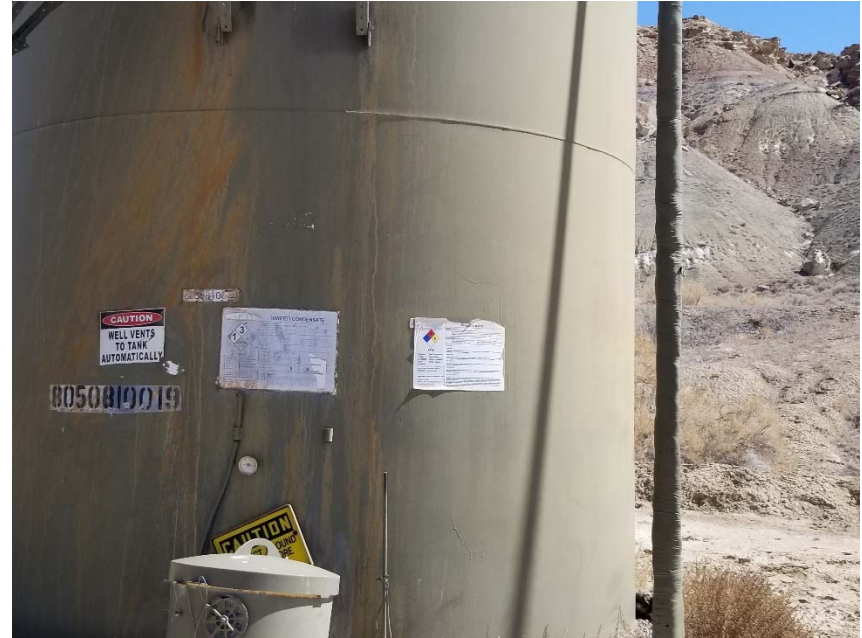
Photo 4. Incomplete tank labels.
