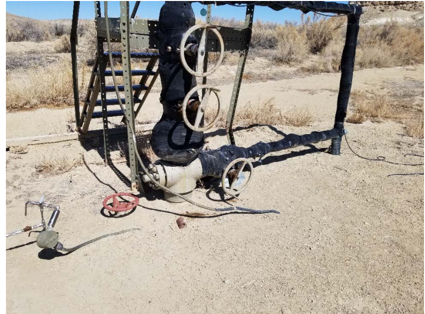
Photo 2. No bradenhead access apparent.
