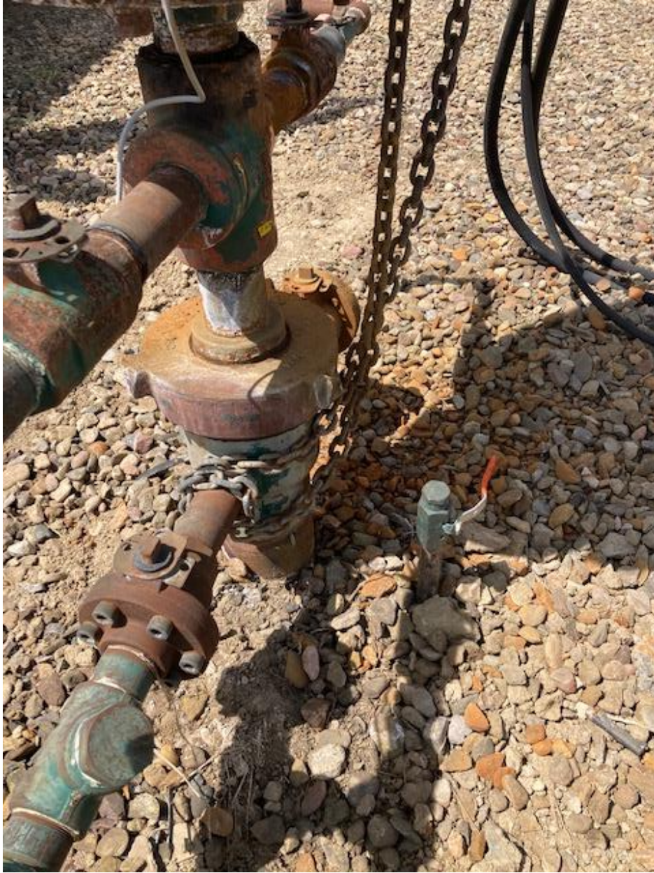
Plumbed Bradenhead to the surface to comply with Rule 341.
