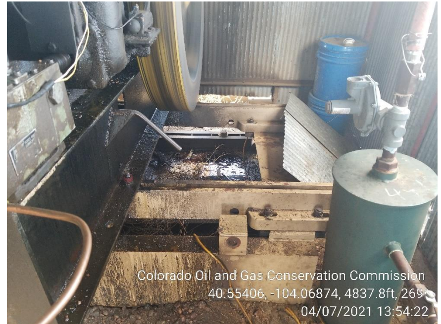
Photo 8 – Stained Soil at Gas Engine
