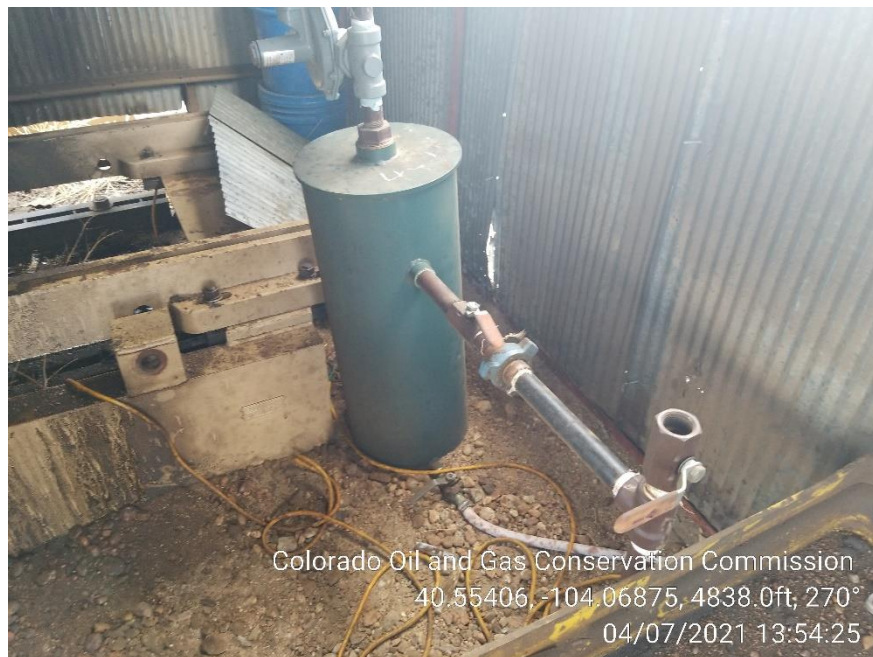
Photo 9 – Stained Soil at Gas Engine
