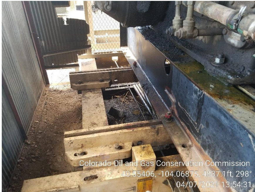
Photo 11 – Stained Soil at Gas Engine
