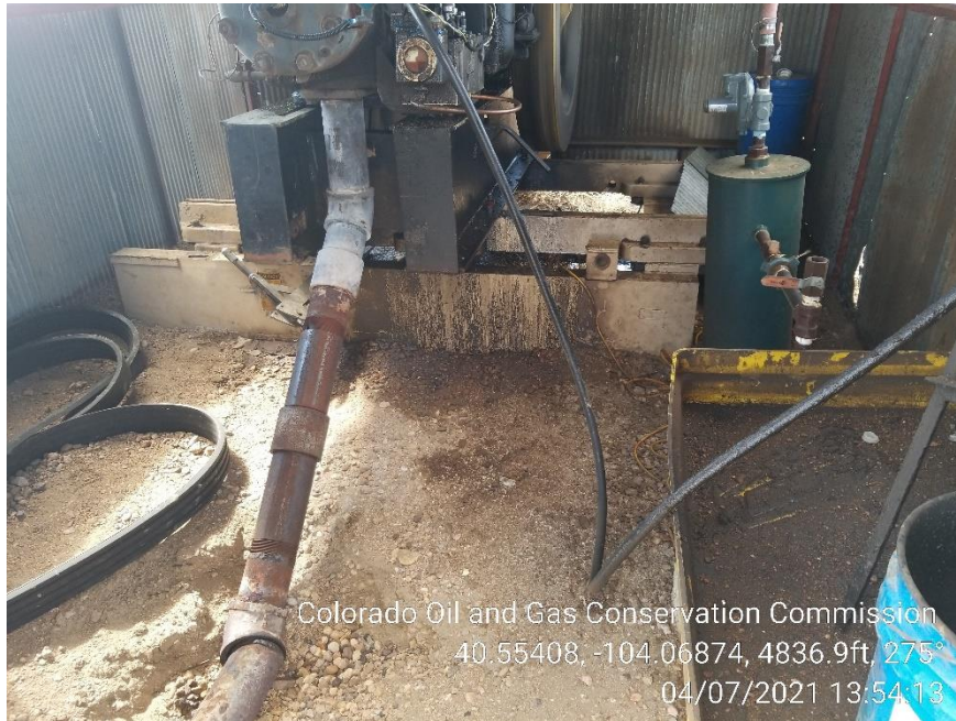
Photo 7 – Stained Soil at Gas Engine
