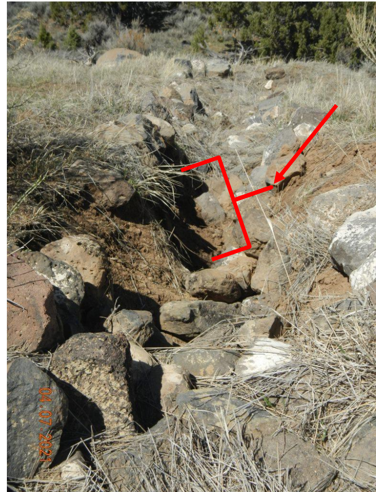
Photo#5: Rocked drain at NE corner. Undercutting area marked with red
