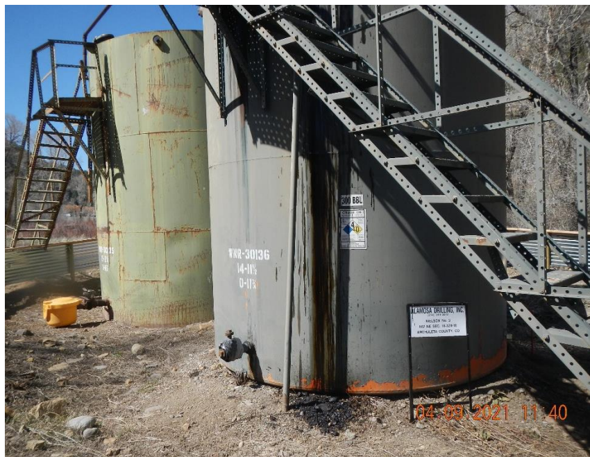
Northern AST has oil staining the side.
