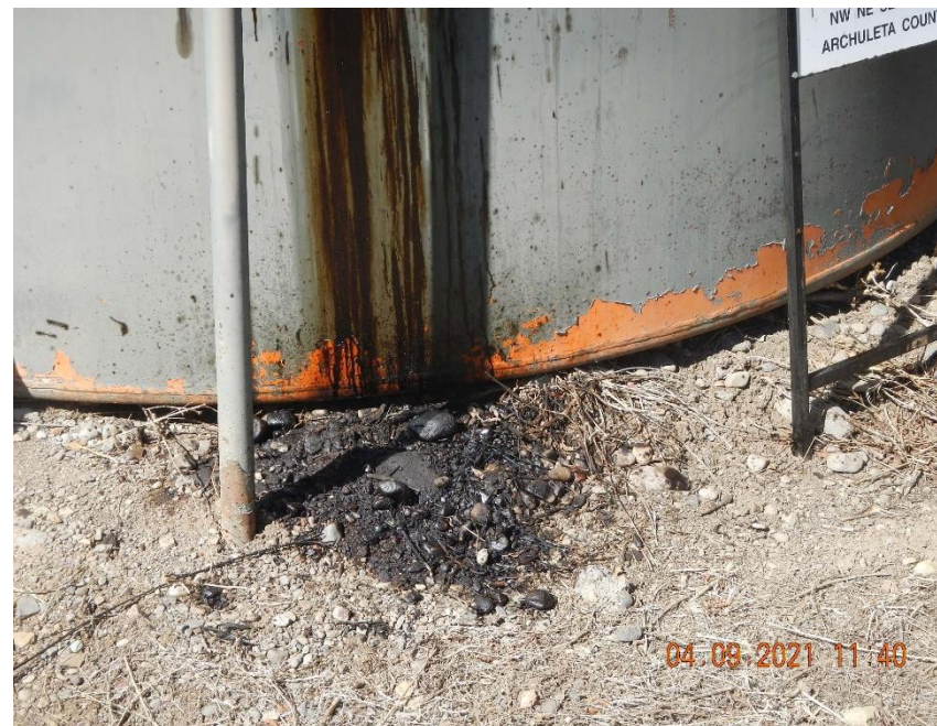
Oil stained soil at the base of the northern AST.
