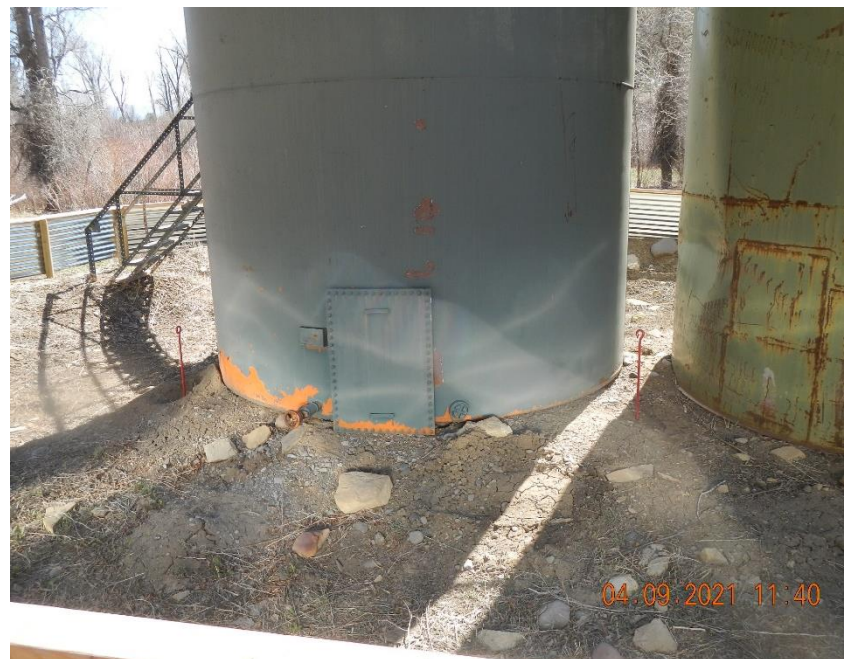
Anchors have been installed, but are not connected to the tanks.
