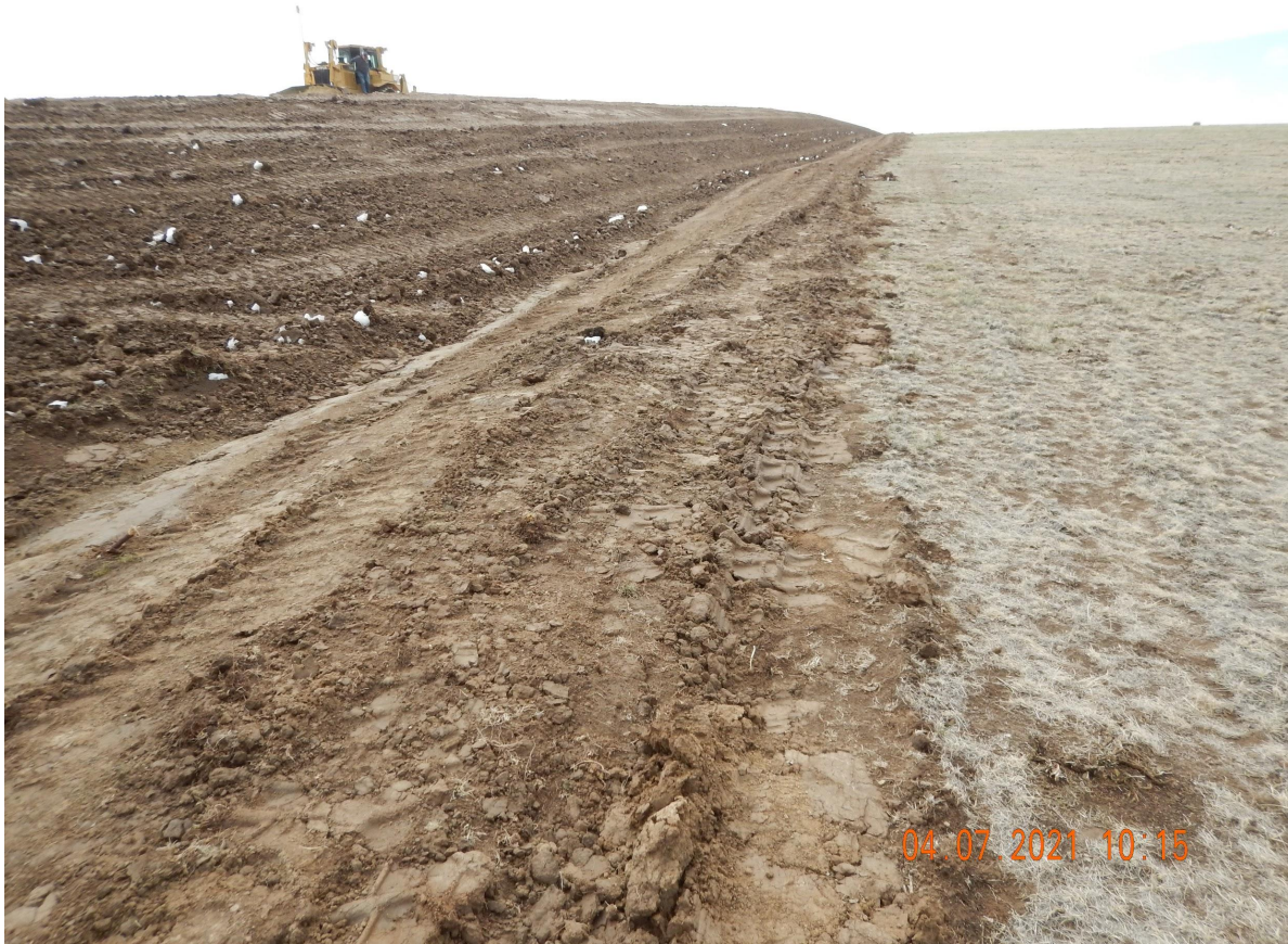
Photo 6. Photo taken from the western location, facing South. Photo illustrates the Operator has sufficiently stabilized the berm BMP.
