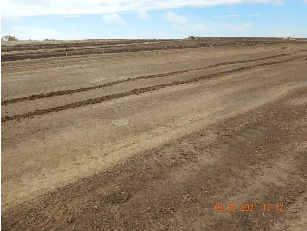
Photo 7. Photo taken from the northern location, facing Southwest. Photo illustrates the Operator appears to have salvaged topsoil in compliance with Rule 1002.b. There was an observed color change from topsoil to subsoil.
