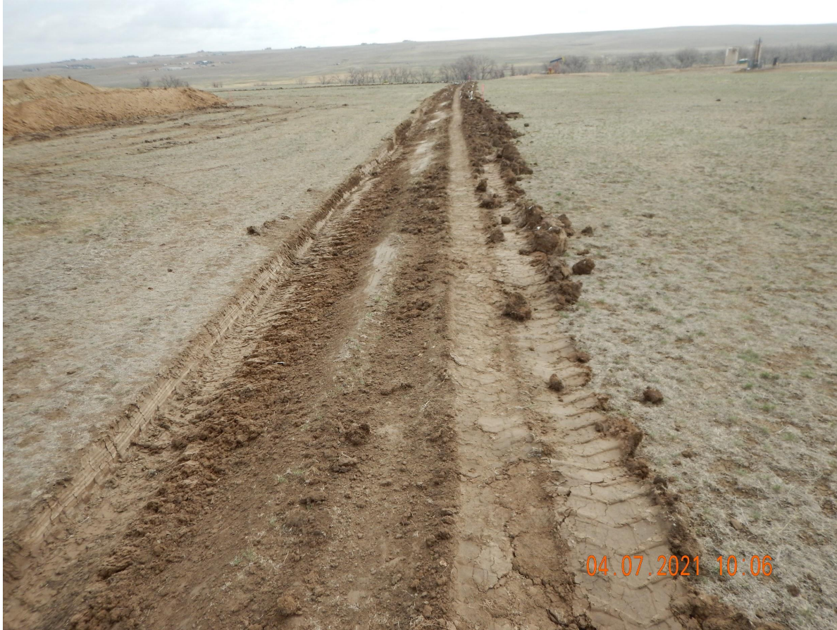
Photo 1. Photo taken from the southern location, facing East. Photo illustrates the Operator has installed a ditch and berm BMP during construction operations. However, the BMP is not in proper functioning condition.
