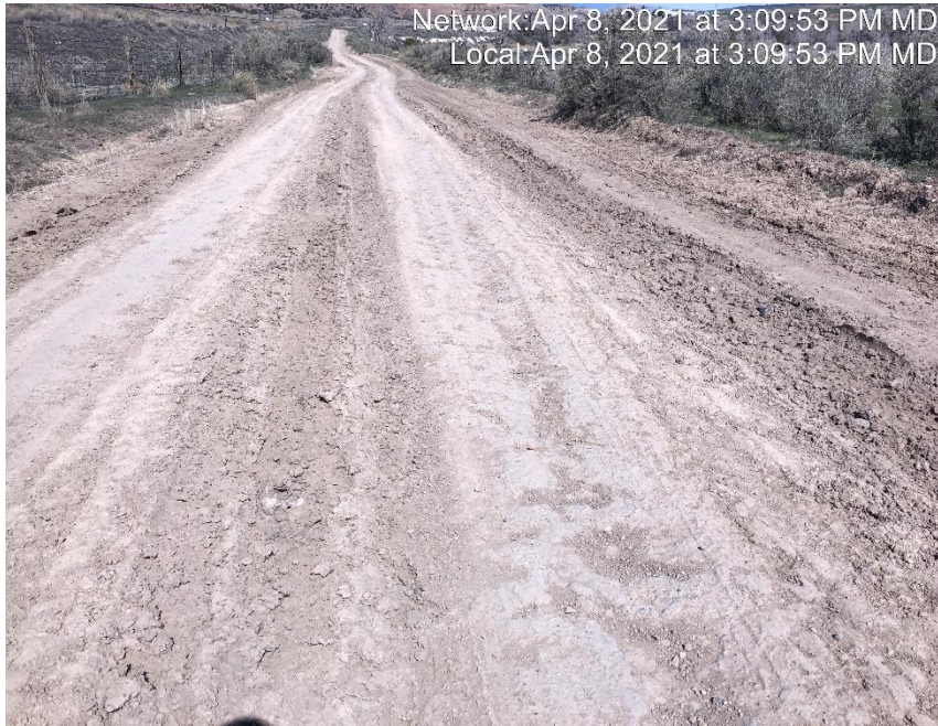
Photo #3439 Access road lacks stabilization
