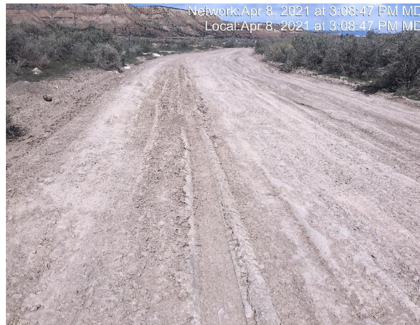
Photo #3438 Access road lacks stabilization
