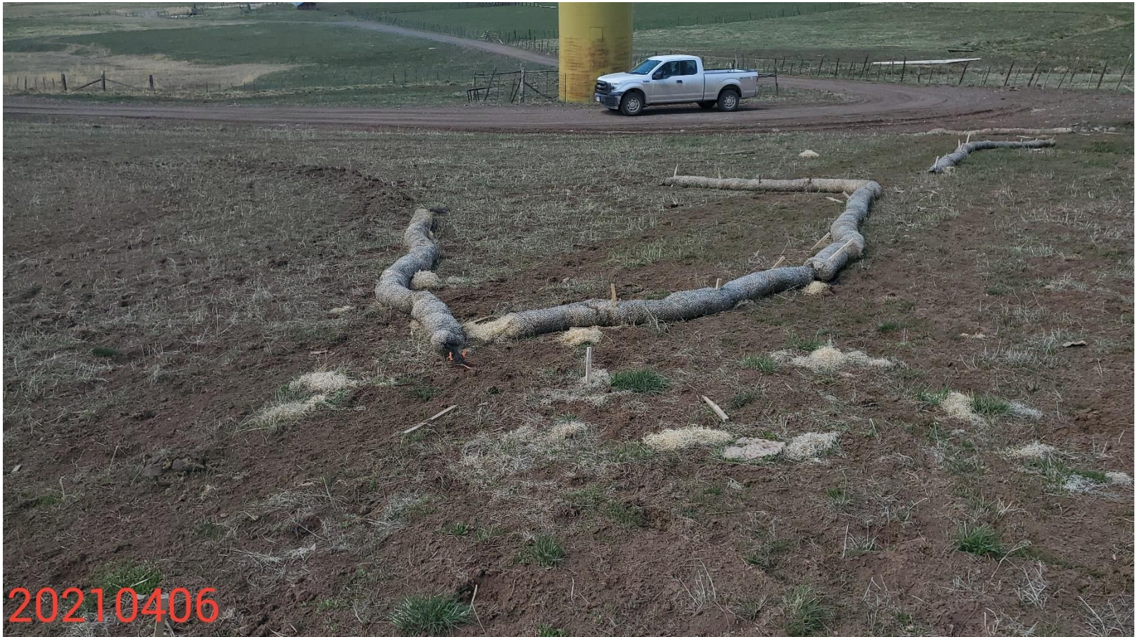
Photo 7: Photo shows straw wattle BMPs have not been maintained in proper functioning condition, is now considered debris and requires removal.
