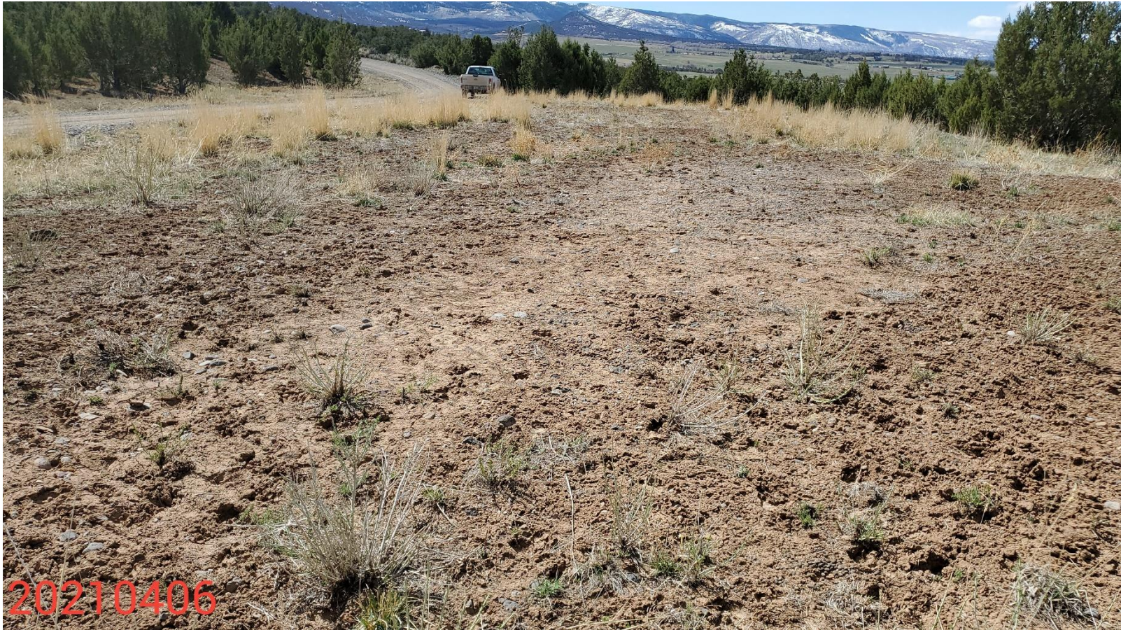
Photo 4: Photo taken from the north end of the Location, facing south. Photo shows large areas of the Location remain bare and graveled. Compaction concerns exist. Unable to find evidence that final reclamation activities have been completed in accordance with 1004 Rules.
