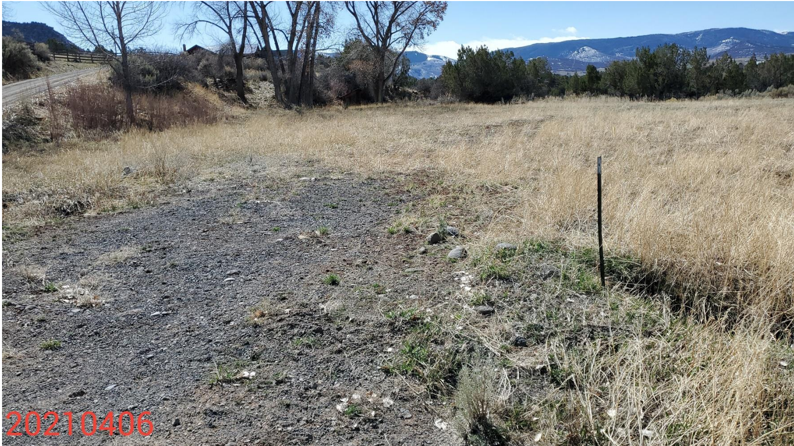
Photo 1: Photo taken from the Location entrance, facing south. Photo shows reclamation has not been conducted in accordance with COGCC 1004 Rules; culvert has not been removed and entrance reclaimed; gravel remaining on the Locaiton.
