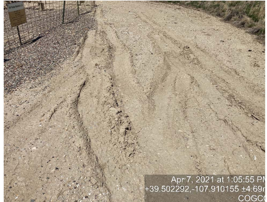
Lack of stabilization/compaction
