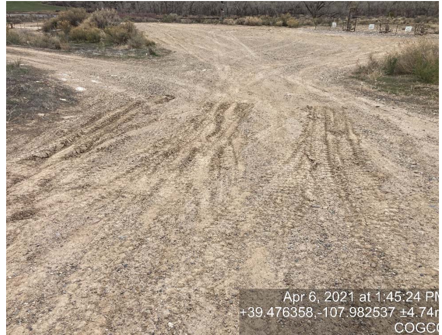
Lack of stabilization/compaction
