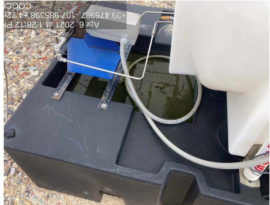
chemical tank containment is full of fluid
