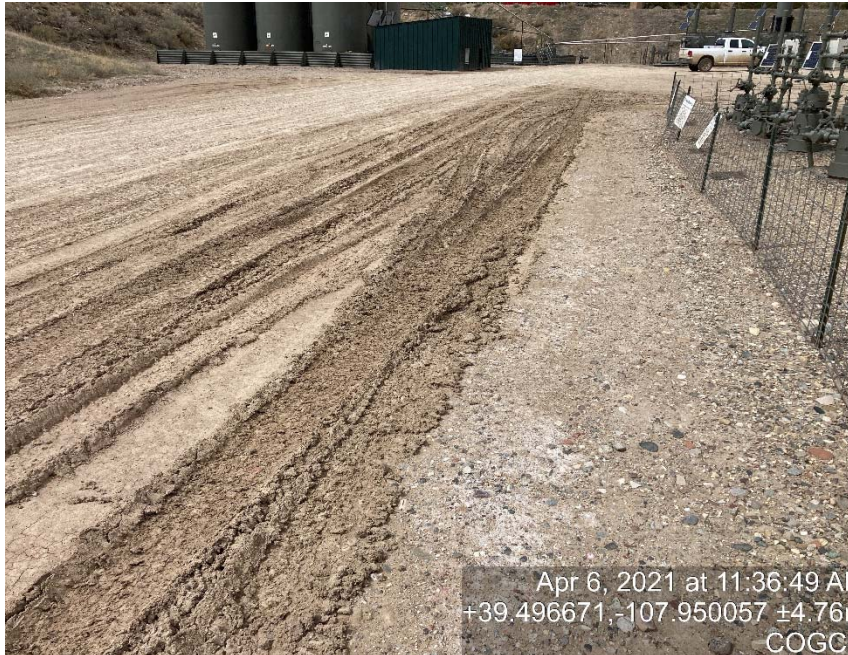
Lack of stabilization/compaction
