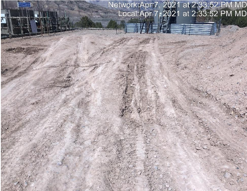
Photo #3402 Location lacks stabilization.
