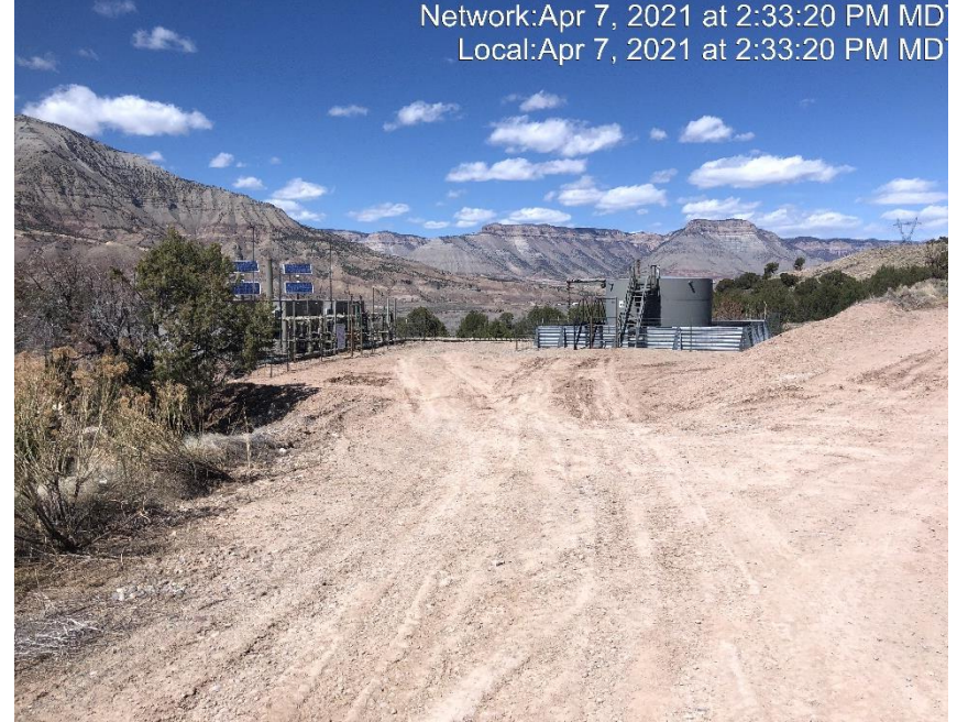
Photo #3401 No form of tracking control at entrance to location.
