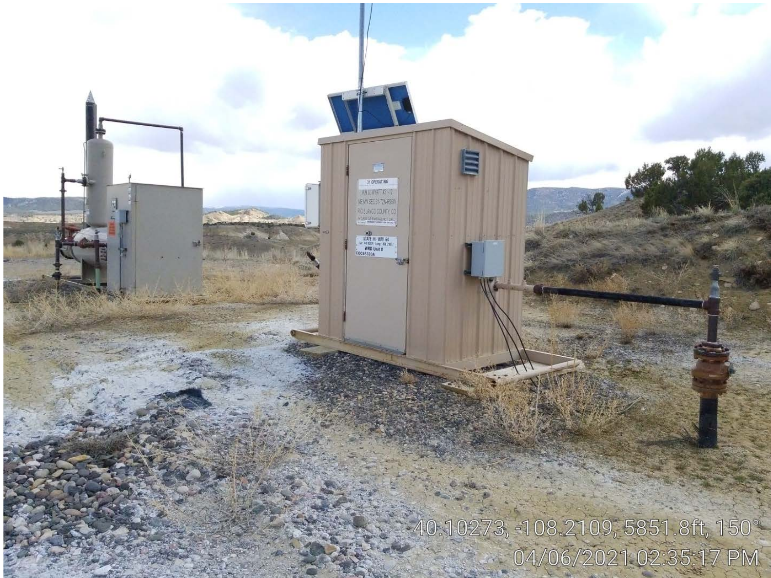
Photo 3. Meter building & separator.
