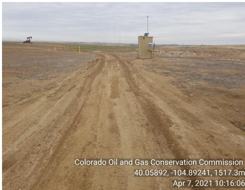
Photo 9 Deep ruts on access road, road in need of proper BMP's
