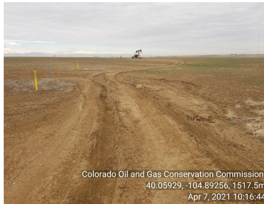
Photo 10 Deep ruts on access road, road in need of proper BMP's
