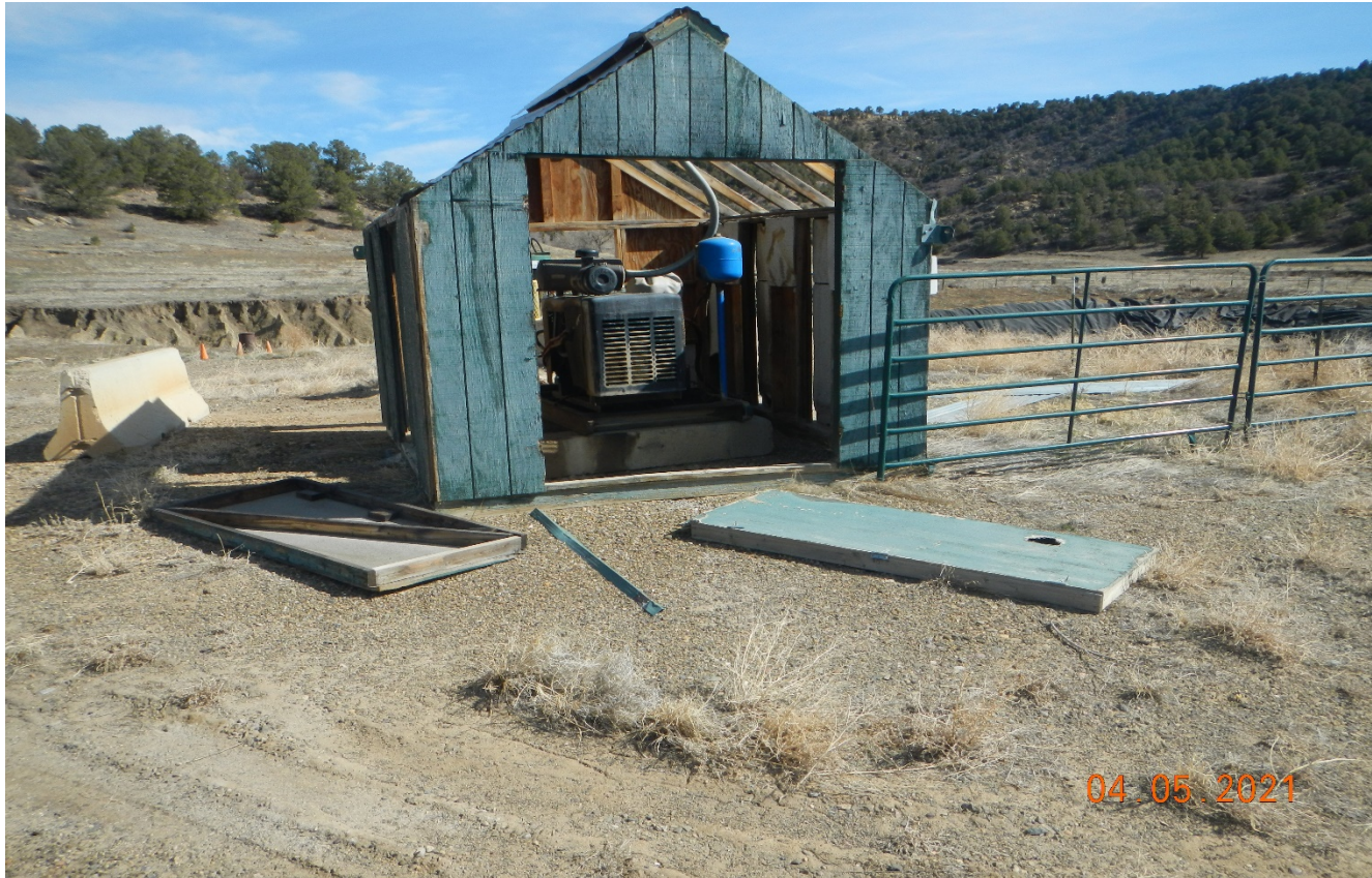
Photo 1. The shed is in disrepair and panels are laying on the ground.
