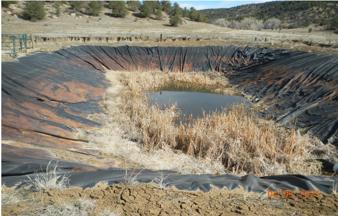
Photo 3. No freeboard marker was observed.
