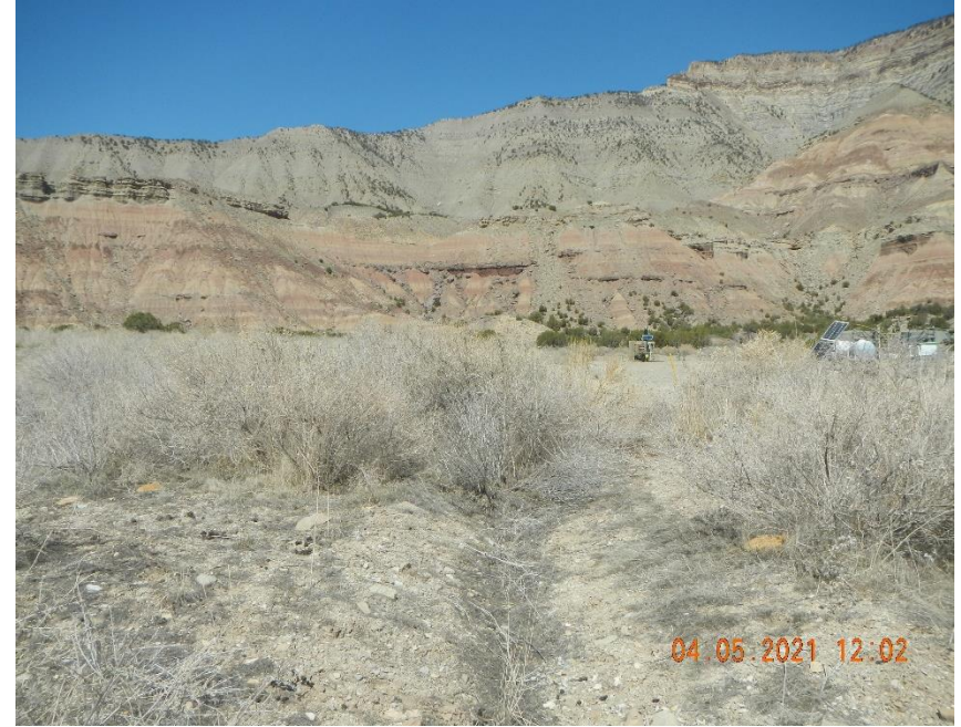
Ditch along west edge of location is clogged sediment trapped by vegetation growing in south west corner of location.
