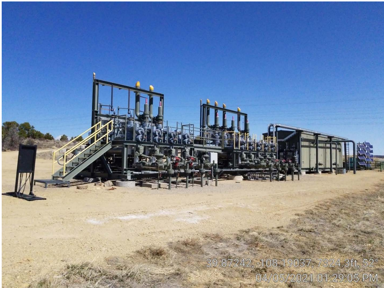
Photo 2. Well manifold & separator.
