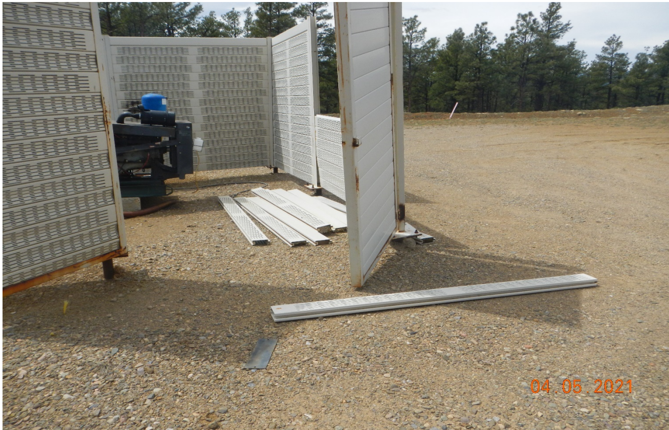
Photo 2. Panels of the sound wall are laying on the ground.
