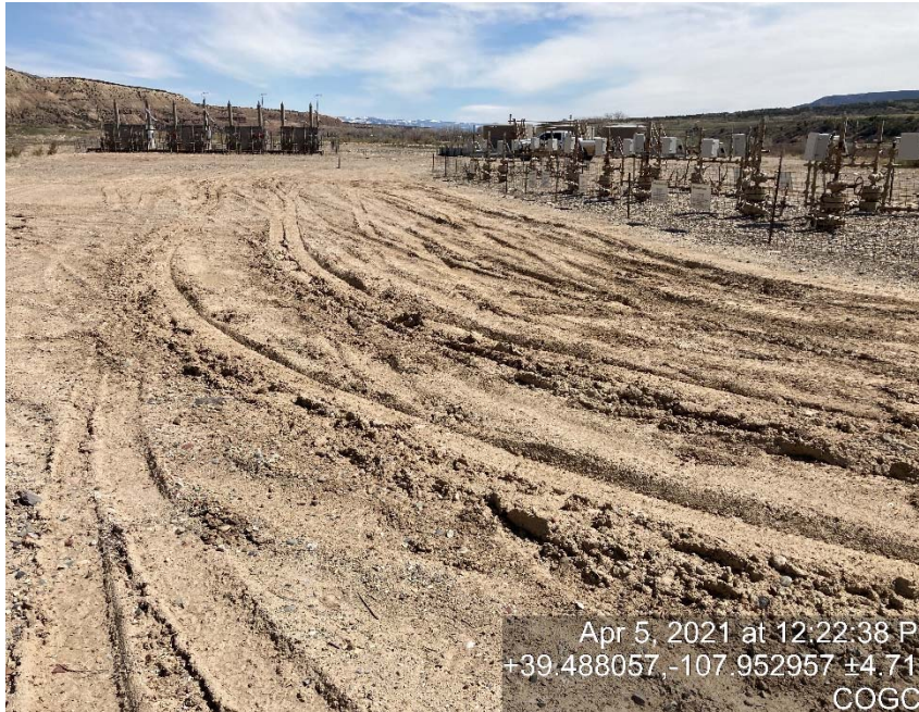
Lack of stabilization/compaction
