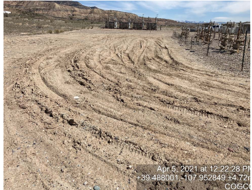
Lack of stabilization/compaction
