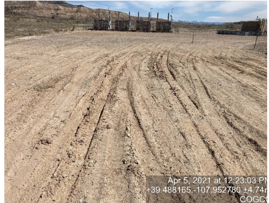
Lack of stabilization/compaction
