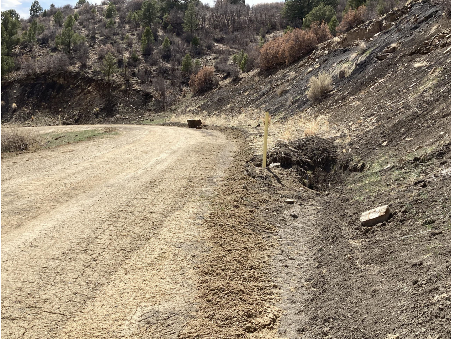
PHOTO 5: THE BAR DITCH WAS DOMINATED TO ALLOW STORMWATER TO FLOW TO THE CULVERT INLETS.
