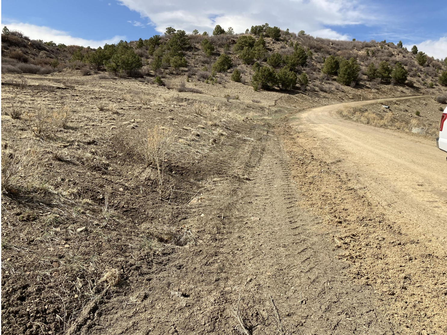
PHOTO 11: THE BAR DITCH WAS BACK FILLED AND THE SOIL WAS COMPACTED WITH THE TIRE OF THE BACKHOE FOR SOIL STABILIZATION AND TO ELIMINATED THE DITCH CUTTING ALONG THE ACCESS ROAD.
