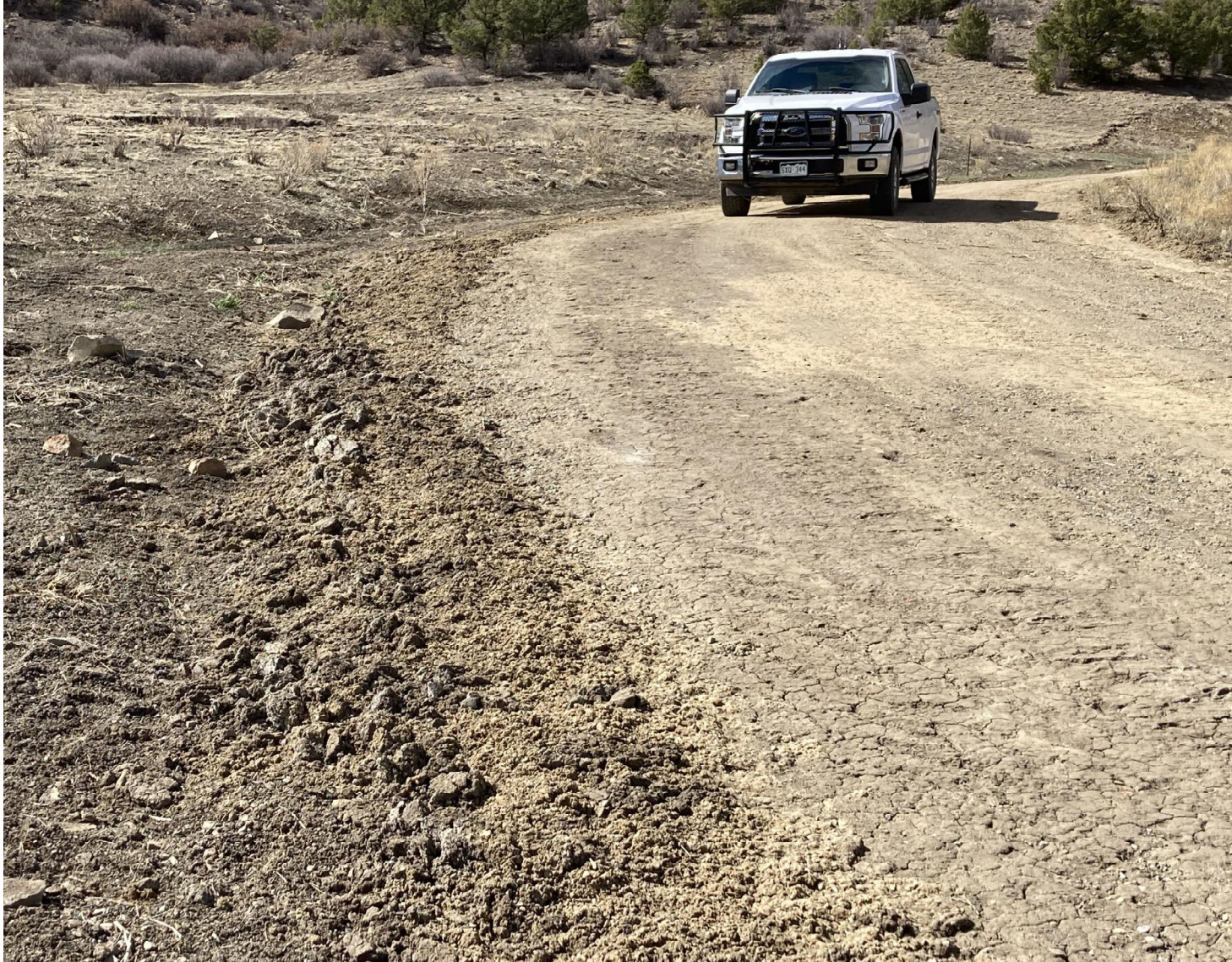
PHOTO 12: THE ACCESS ROAD WAS SURFACE CROWNED TO ESTABLISH SHEET FLOW AND ELIMINATE THE CHANNELIZED AREAS OF THE ROAD SURFACE.
