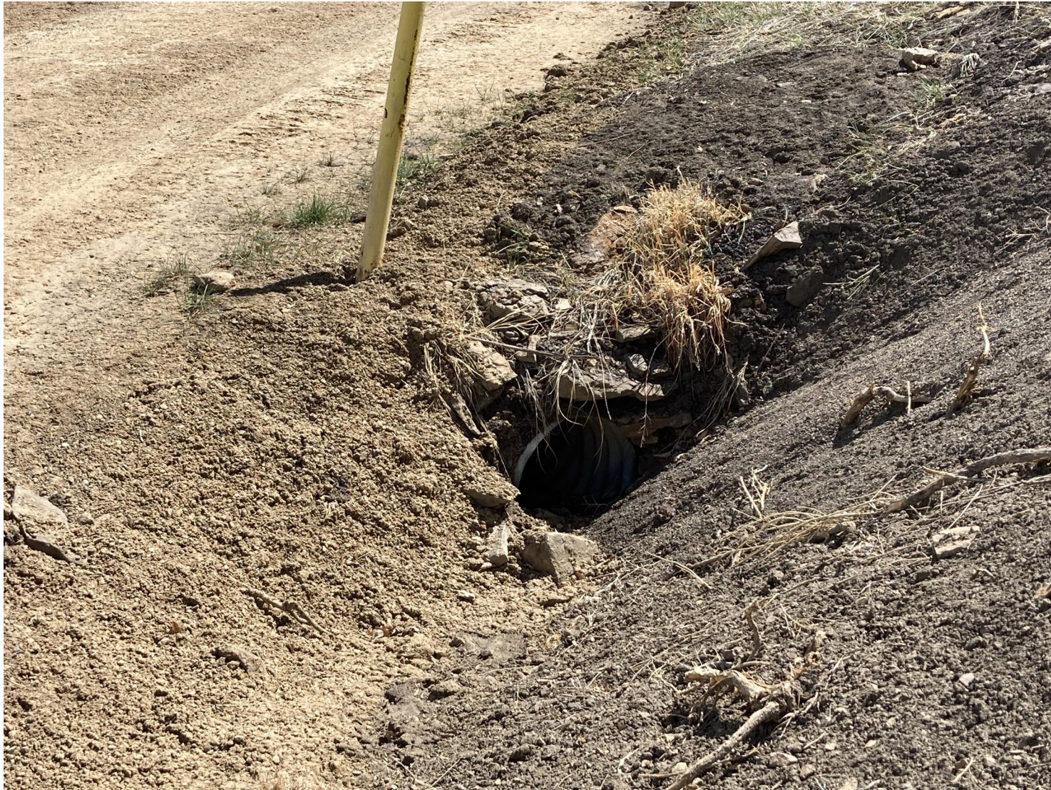
PHOTO 7: THE SEDIMENT ACCUMULATION WAS REMOVED FROM THE CULVERT INLET.
