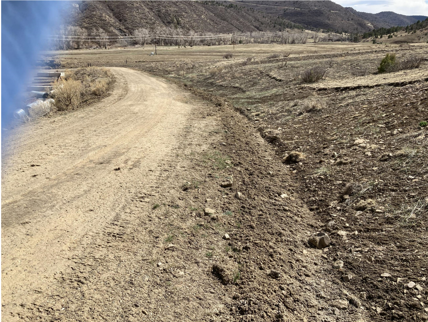
PHOTO 10: THE ACCESS ROAD WAS SURFACE CROWNED TO ESTABLISH SHEET FLOW AND ELIMINATE THE CHANNELIZED AREAS OF THE ROAD SURFACE.
