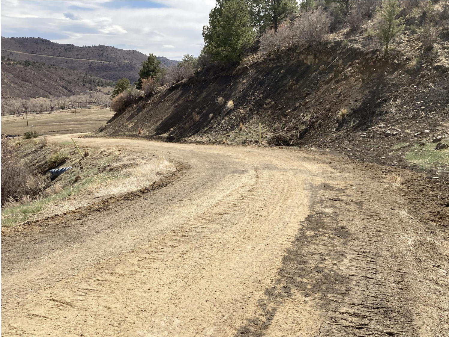
PHOTO 8: THE ACCESS ROAD WAS SURFACE CROWNED TO ESTABLISH SHEET FLOW AND ELIMINATE THE CHANNELIZED AREAS OF THE ROAD SURFACE. THE BAR DITCH WAS DOMINATED TO RECEIVE STORMWATER.
