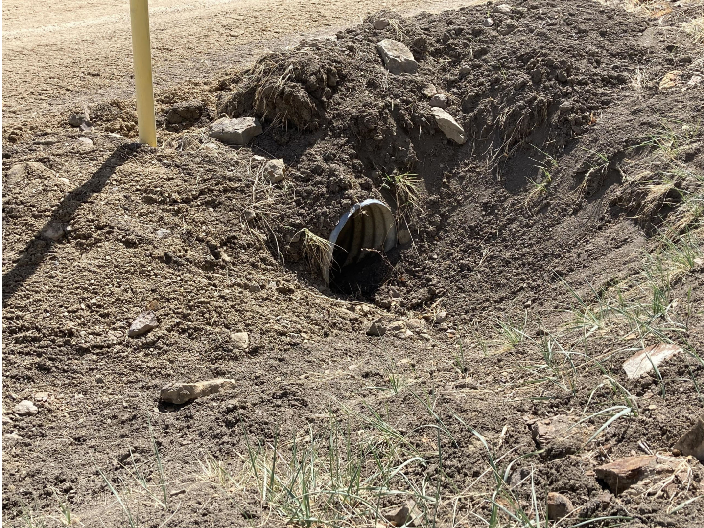
PHOTO 6: THE SEDIMENT ACCUMULATION WAS REMOVED FROM THE CULVERT INLET.
