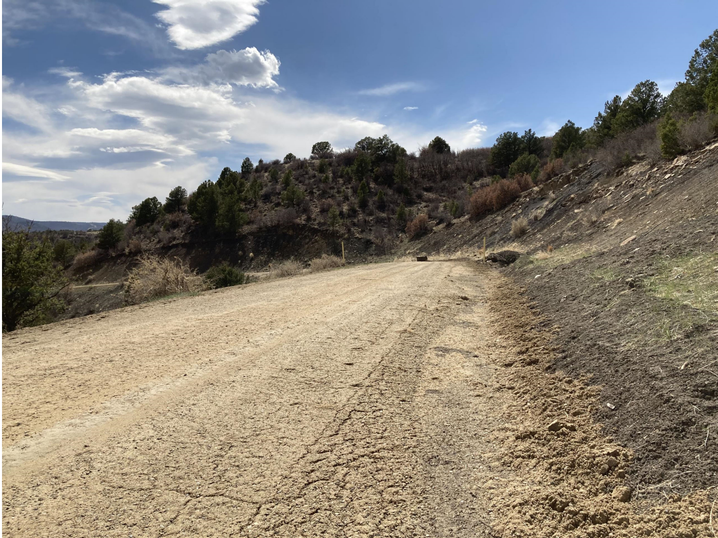
PHOTO 4: THE SEDIMENT ACCUMULATION AND VEGETATION WAS REMOVED FROM THE BAR DITCH TO RECEIVE RUN OFF FROM THE ACCESS ROAD.
