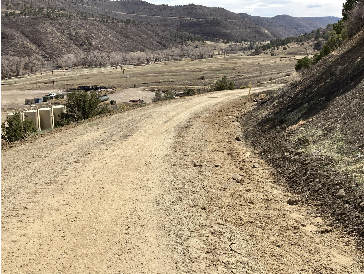
PHOTO 9: THE ACCESS ROAD WAS SURFACE CROWNED TO ESTABLISH SHEET FLOW AND ELIMINATE THE CHANNELIZED AREAS OF THE ROAD SURFACE. RUN OFF IS DIRECTED TO THE CULVERT INLETS.
