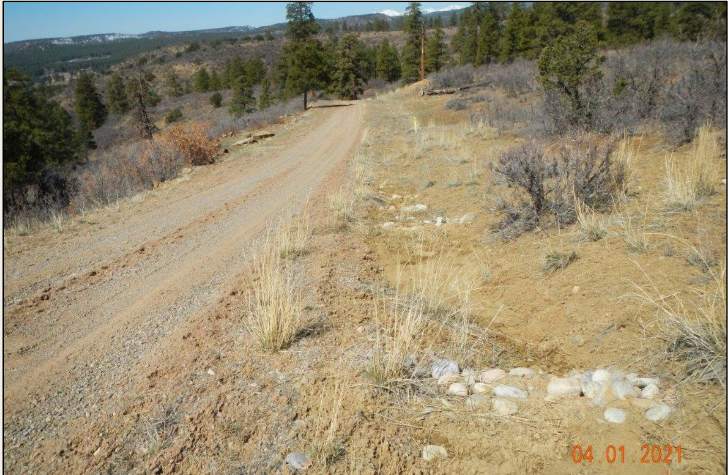
Photo 4. View of velocity checks at the bottom of the slope that are full of sediment and overflowing. These need maintenance.
