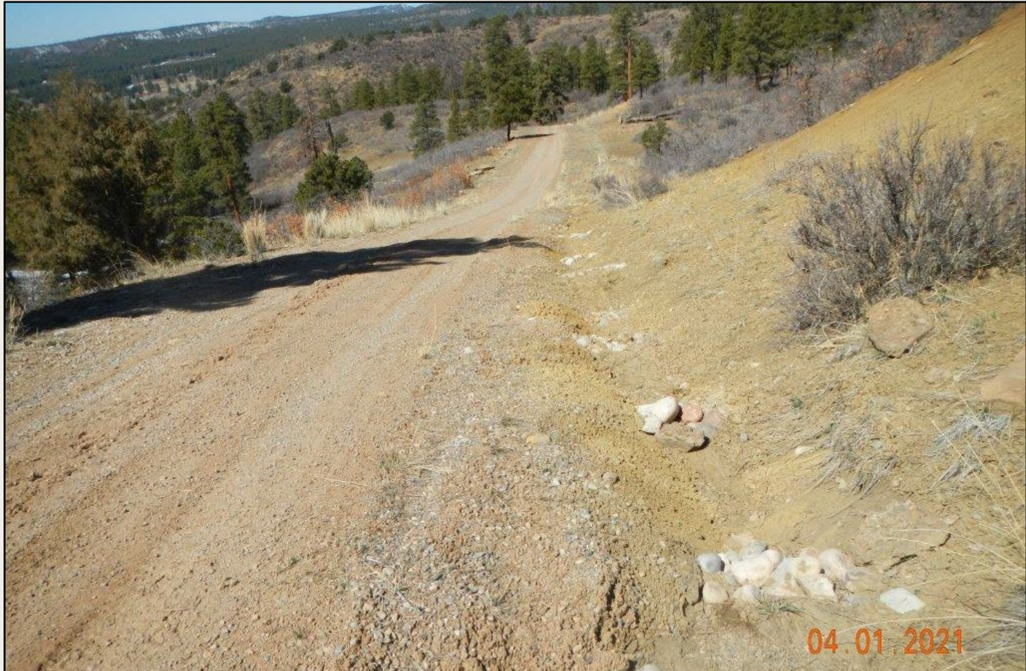
Photo 3. View of velocity checks placed along the access road. These checks are not properly sized/installed as stormwater flows around the checks resulting in continued erosion along the roadside.
