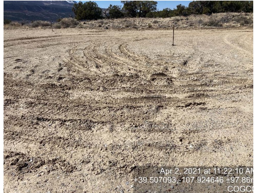
Lack of stabilization/compaction
