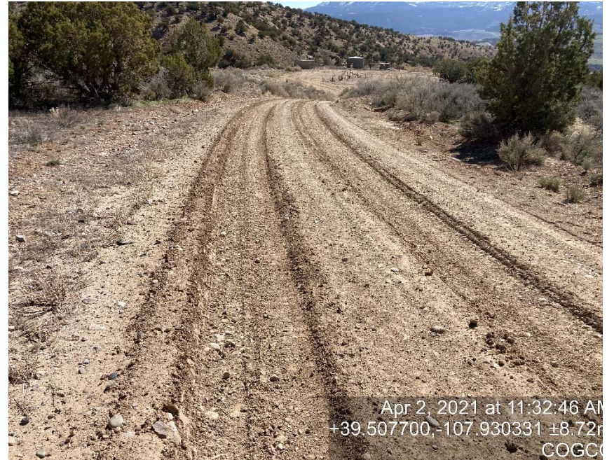
Lack of stabilization/compaction
