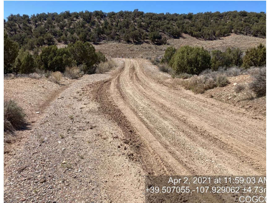
location entrance access road/Lack of stabilization/compaction
