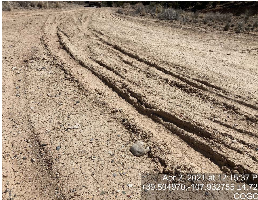
Lack of stabilization/compaction
